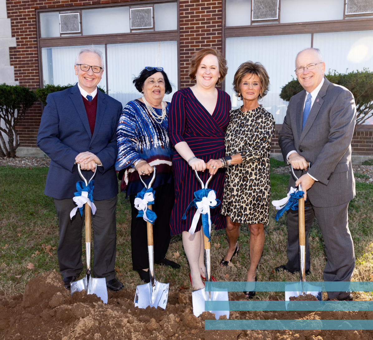
The groundbreaking for the Terry L. “Bo” Pace Advanced Welding and Fabrication Technology Program was held Dec. 1, 2021.
