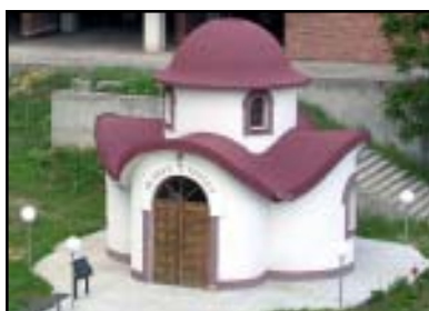
The University chapel and new library, which is under construction.
